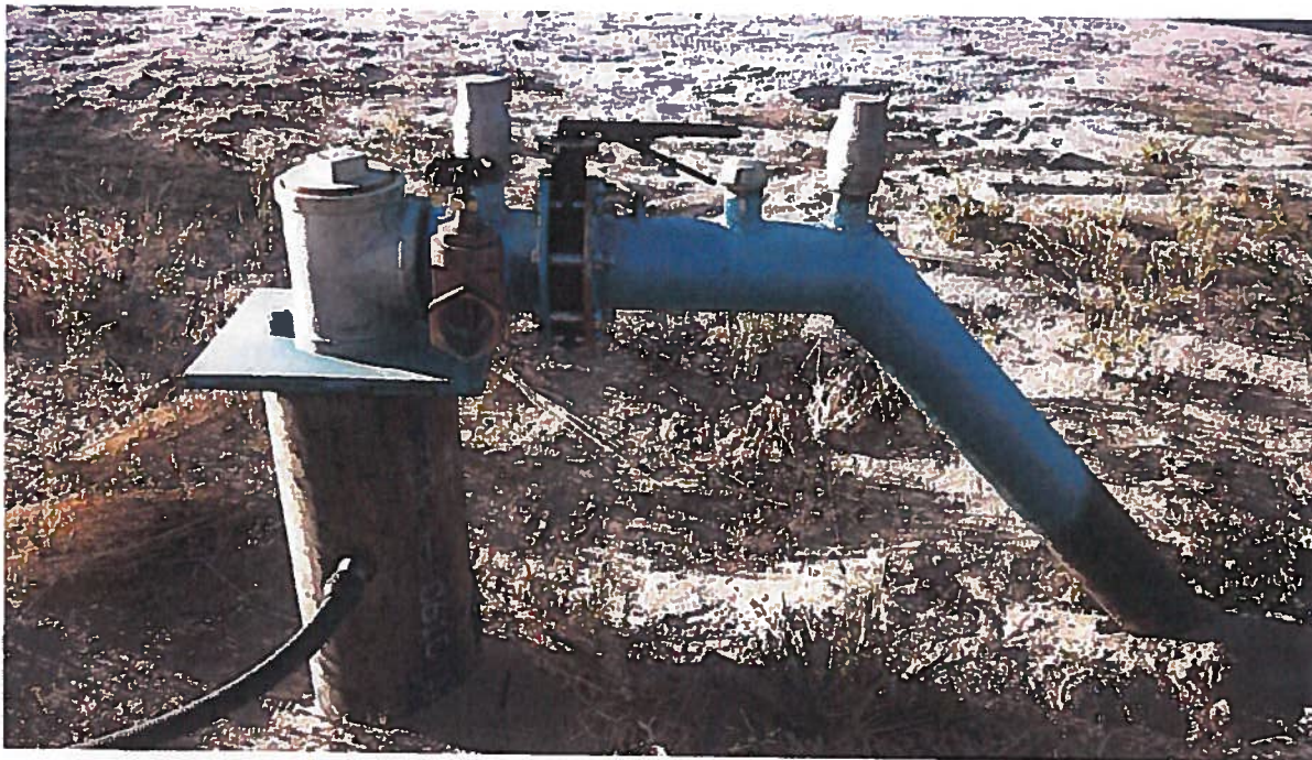
Photo 1. View of POD.
