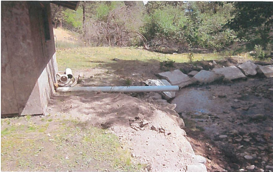
Discharge of water from powerhouse to Robie Creek.
