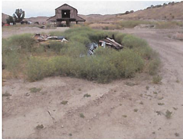
Piping from old system
