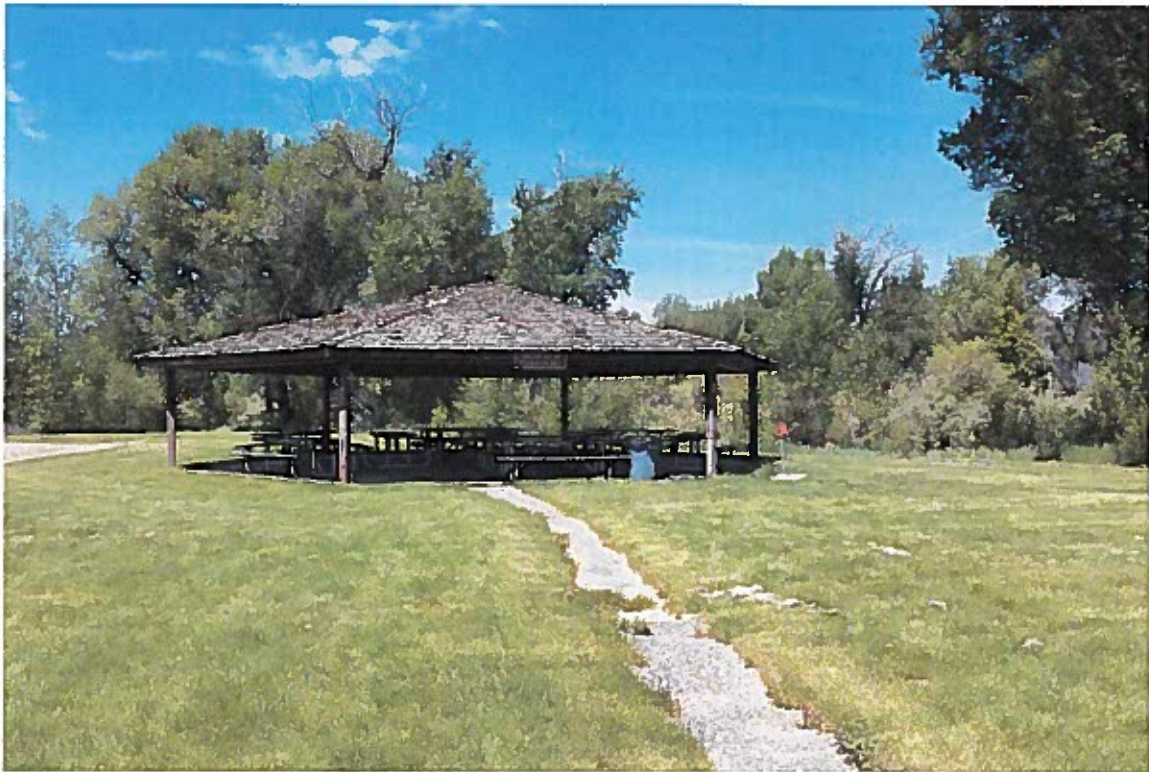
Typical Large Picnic Shelter
