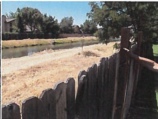
Headgate and concrete box from top of wooden box
