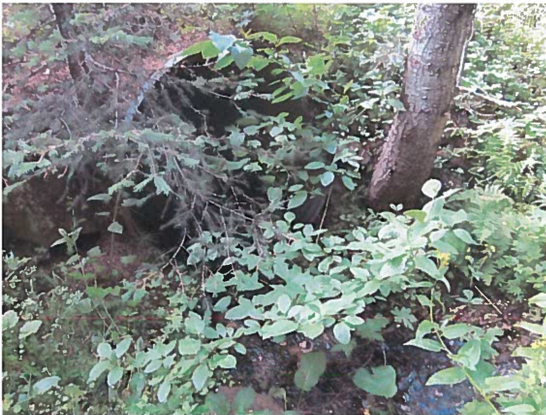
12. Looking downstream on connection ditch just above Anderson Reservoir Road. This culvert is the same as shown in picture #10.
