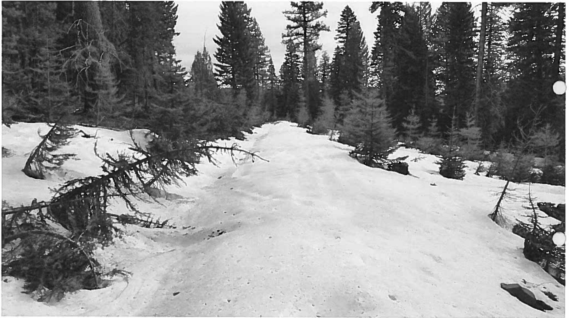
Seawell Creek Ditch Looking up ditch about a half mile from Seawell Creek May 05 2016
