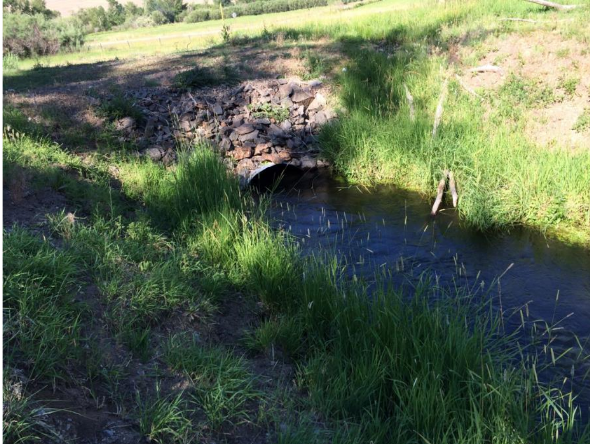
Looking south at the same culvert.
