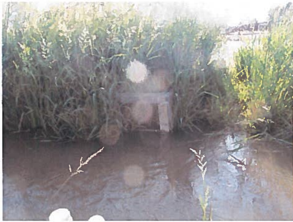
Piping on East side of Eight Mile Creek
