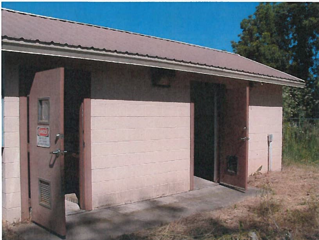
JD Well House - Room on left is chlorination room - Room on right is motor controls and valves.
