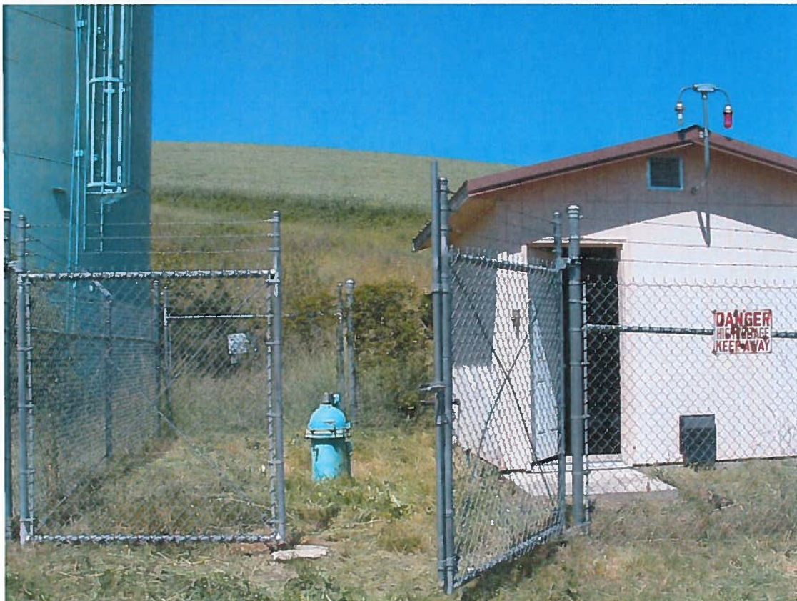
Well 5 with well house on right and 250,000-gallon tank on left
