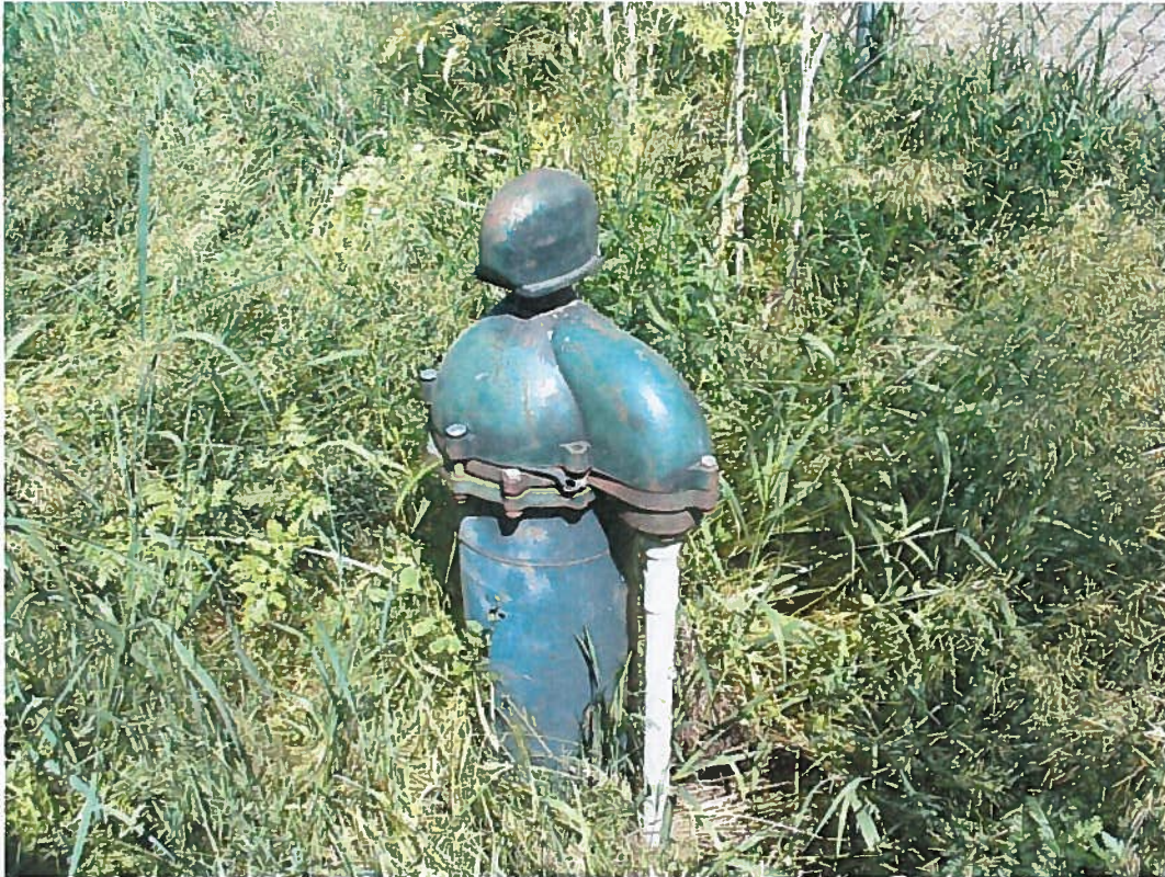
JD Well - Casing and cap; well is located a few feet northwest of the well house
