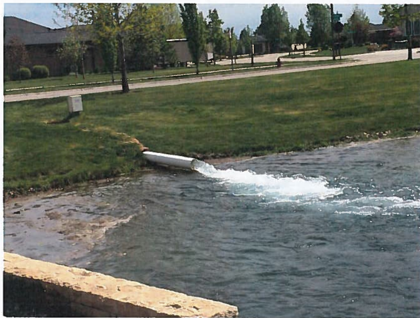
Figure 5. Supply pipe into Pond 2, looking approx. south
