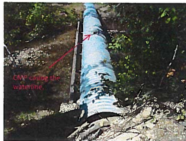
Photo 2. Pipeline crossing Fish Haven Creek.
