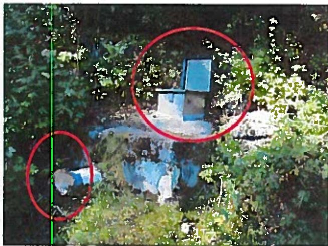
Photo 1. Fish Haven Spring. Overflow is not screened, and lid is not of the proper height.
