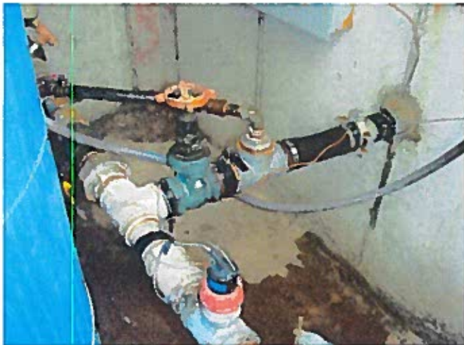
Photo 11. Inside view of the well vault.
