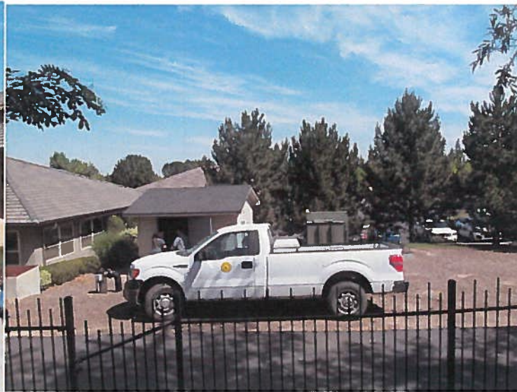
Well house from canal access road
