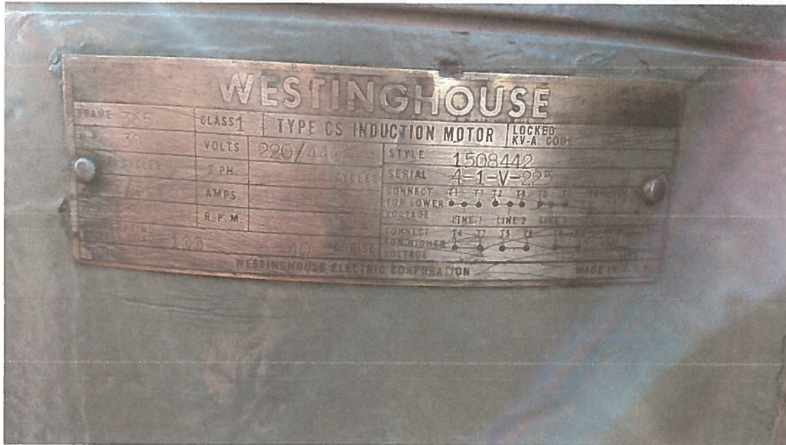
Well #1 motor name plate
