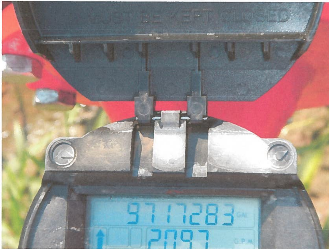
Discharge from new well of 209.7gpm 7-24-2015
