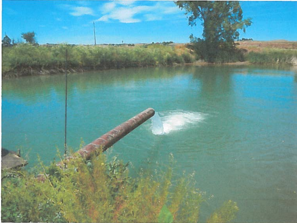
Open discharge from old wells into pumping pond
