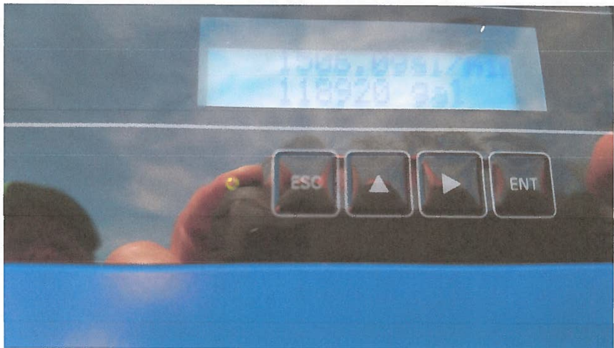
Discharge from old wells of 1,506 gpm 6-3-2016
