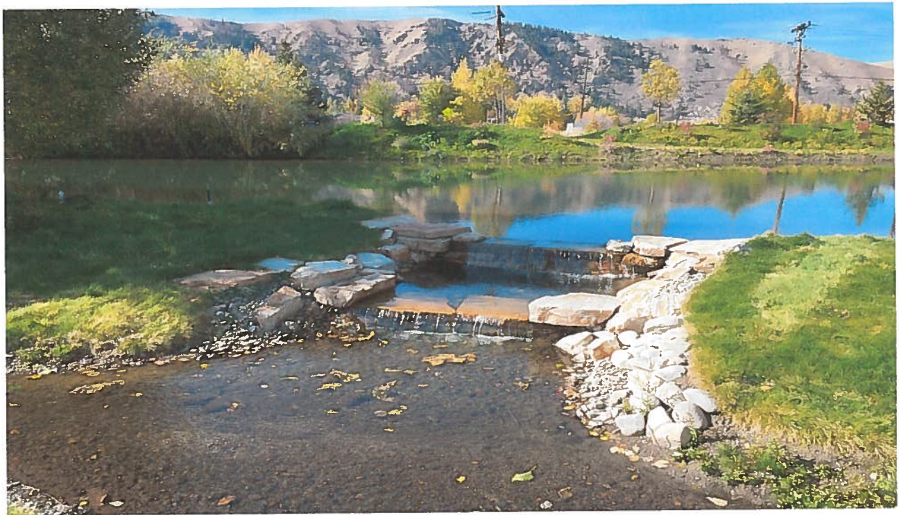
Pond Overflow Outlet
