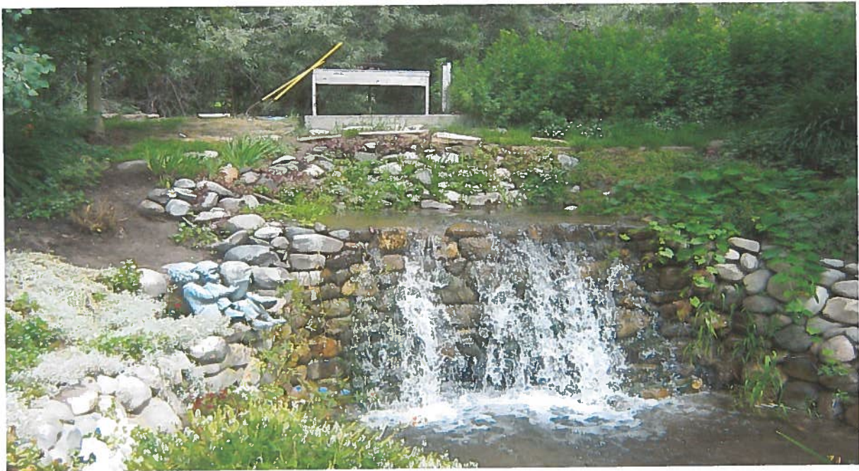
Diversion Structure Hiawatha Canal to Lateral
