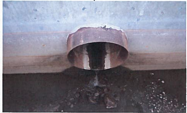
Outlet pipe into concrete dissipater box (from Dam Safety Record)
