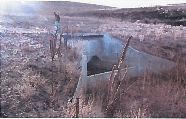
Outlet pipe structure (from Dam Safety Record)
