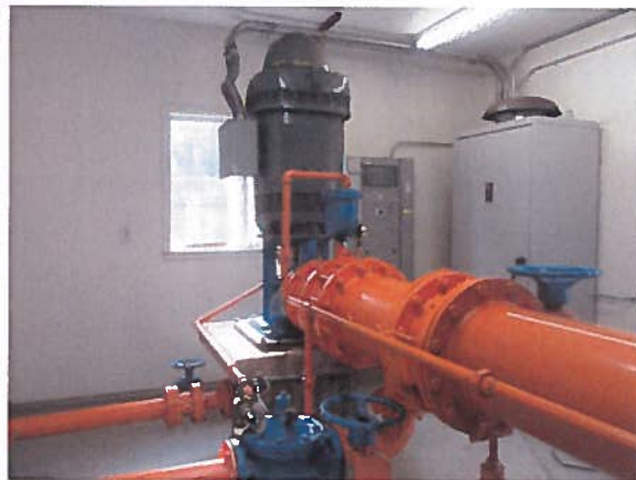
Well No. 6: This well (250 hP) is located at the SE corner of W. State Street and S. Payette Way, near the entrance to Pine Ridge subdivision. The US Electric motor was running at the time of the exam, and the Layne brand pump was producing 1000 gpm (2.23 cfs).
