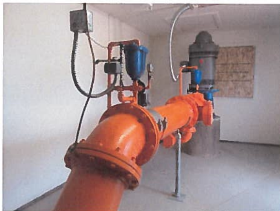
Well No. 7: Well No. 7 is only about 1,500 feet southeast of Well No. 8; it is very close to the Boise River. At the time of the exam, the 200 hP American Marsh pump was on and delivering water to the distribution system.
