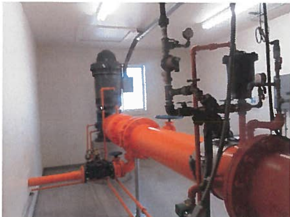
Well No. 8: Well No. 8 (250 hP) is located on S. Anaconda Avenue, only 1,200 feet from the Boise River. The well house looked new and appeared to be designed to blend well with its future residential neighbors. The flow measurement of the American Marsh pump was only diverting about 300 gpm (0.67 cfs).
