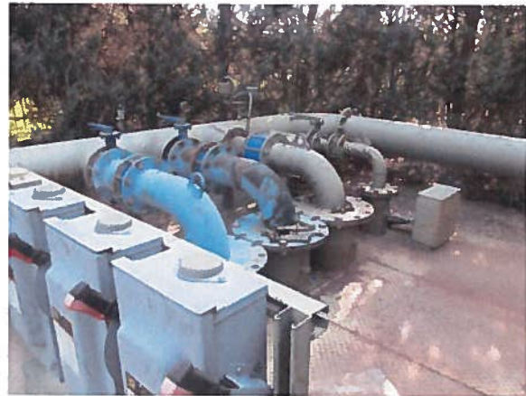
The irrigation pump system (right) utilizes surface water filters and a subsurface vault (left) to clean and pressurize surface water for irrigation.
