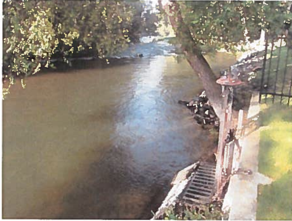
The headgate (left) for water associated with 63-194 enters the buried Mace-Catlin ditch at a location on the Boise River within Island Woods Subdivision. A "weir vault" (right) has been installed immediately following the headgate.
