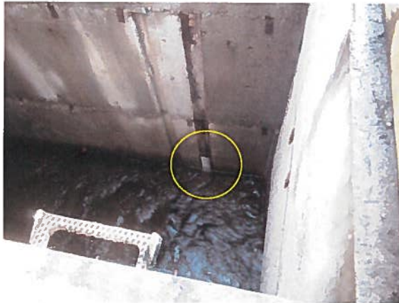
The vault contains a staff gauge (left) for the Dist 63 watermaster to determine the flow delivered to Two Rivers Subdivision. Crossing Eagle Road westward, the surface water is introduced into Two Rivers' clubhouse pond (right).
