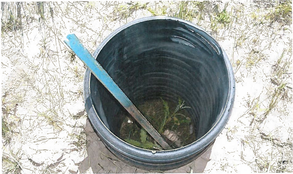
Exposed curb stop at lot.
