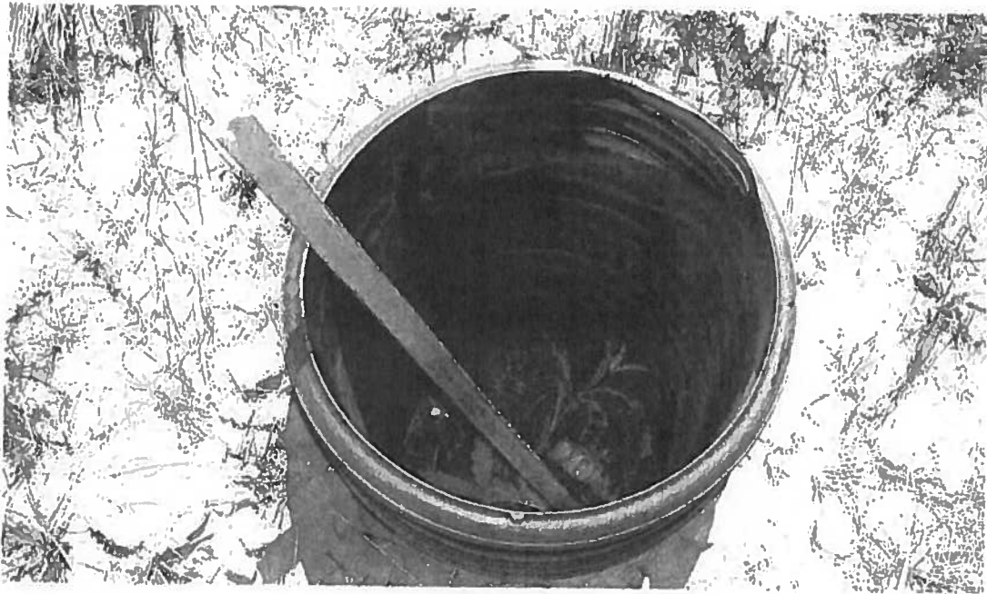
Exposed curb stop at lot.
