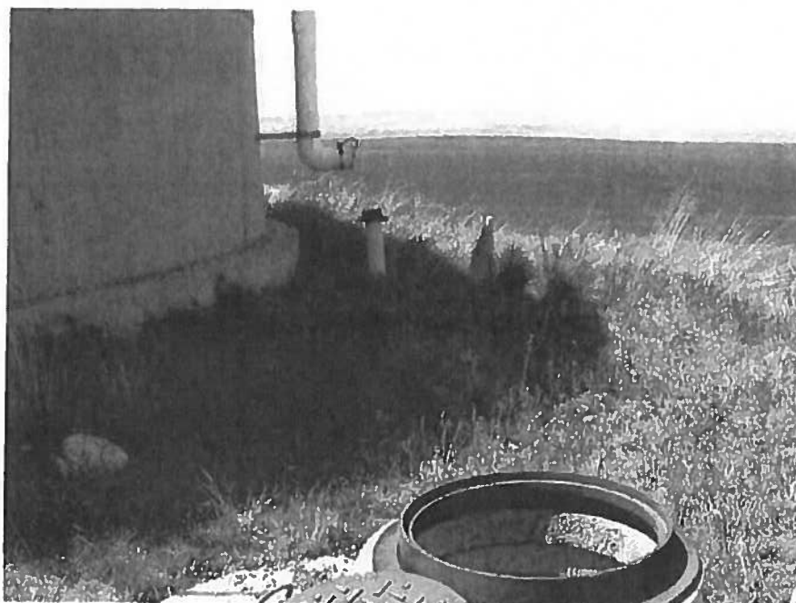
Storage tank showing overflow pipe and valve vault. Water from the wells enters at the top of the tank, then exits the bottom of the tank to the valve vault. Water from valve vault can flow back into delivery pipe when well pumps are off. A tee in the delivery pipe is connected to booster pump. A check valve in valve vault prevents short-circuiting of flow to tank when well pumps are running.
