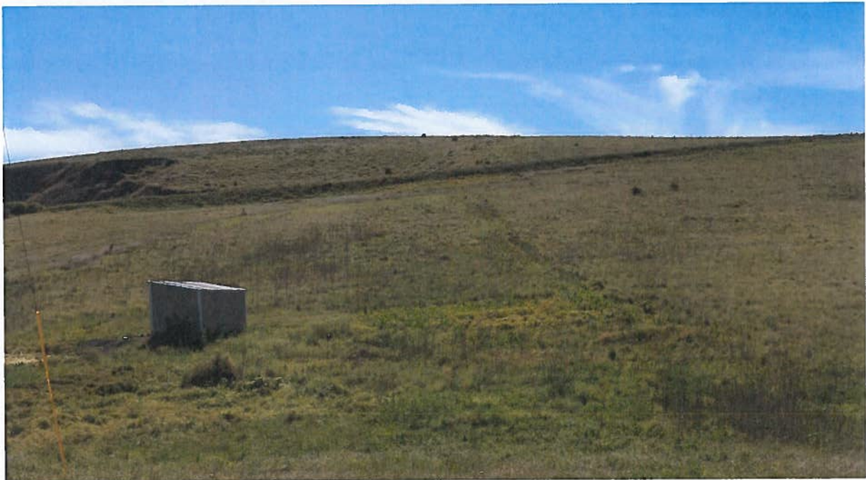
Well house viewed from Powell Road. Scar from pipe trench barely visible extending up hill to road cut.
