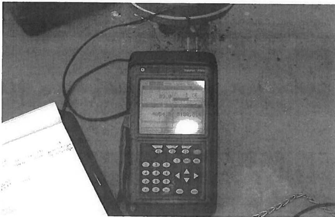
North Well flow rate is 39 gpm with ultrasonic meter and 41 gpm with Neptune turbine meter; 140 psi discharge pressure.
