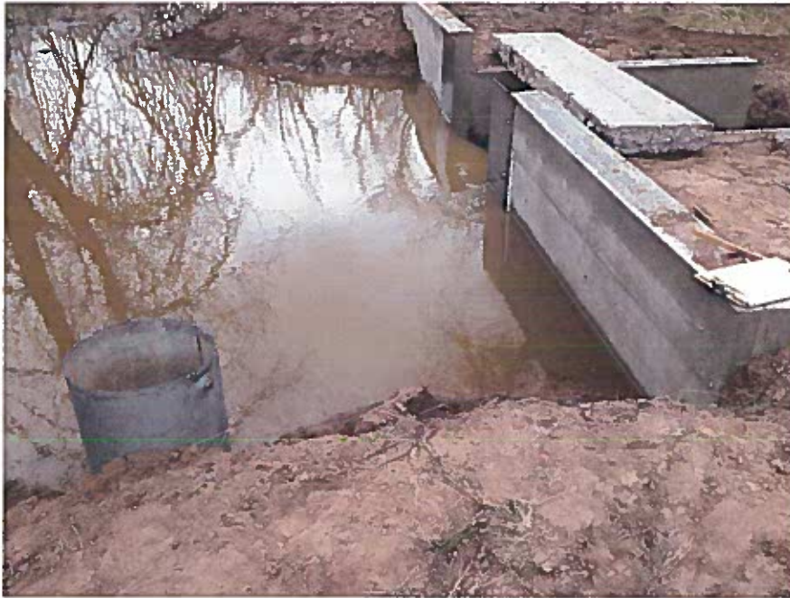
Figure 3: 5' Rectangular Weir with staff gauge on ditch
