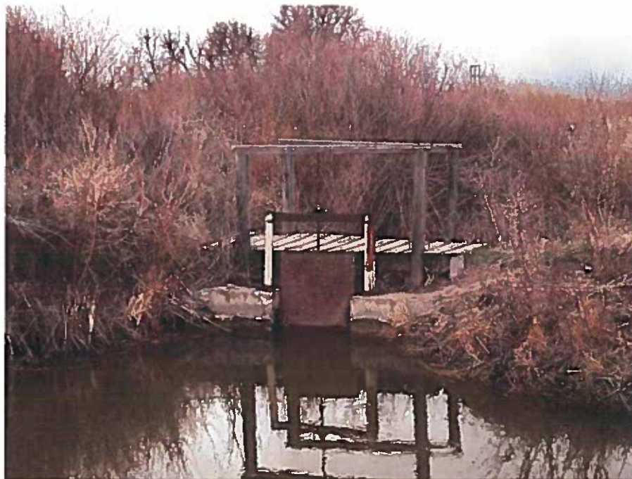
Figure 2: POD from W-Drain into ditch
