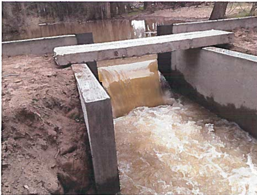
Figure 4: Downstream side of weir
