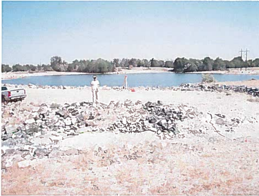
Figure 1: Malad Reservoir from southwest looking north east (2008)
