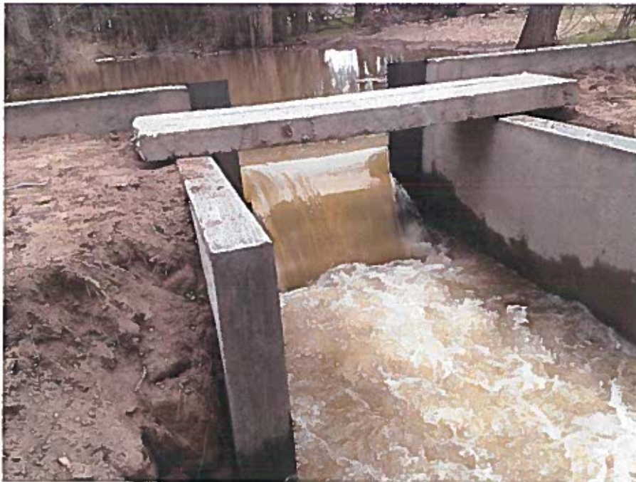
Figure 4: Downstream side of weir
