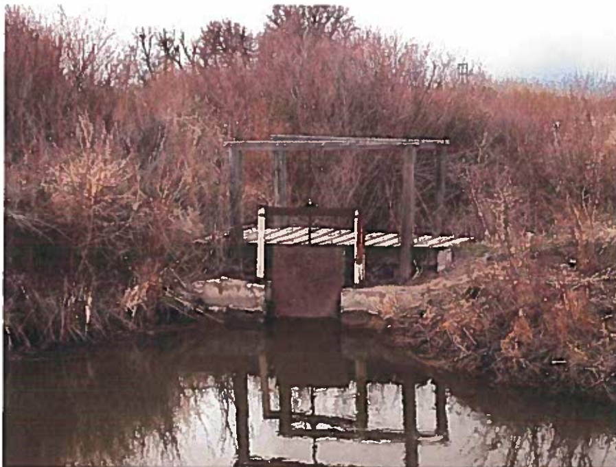
Figure 2: POD from W-Drain into ditch
