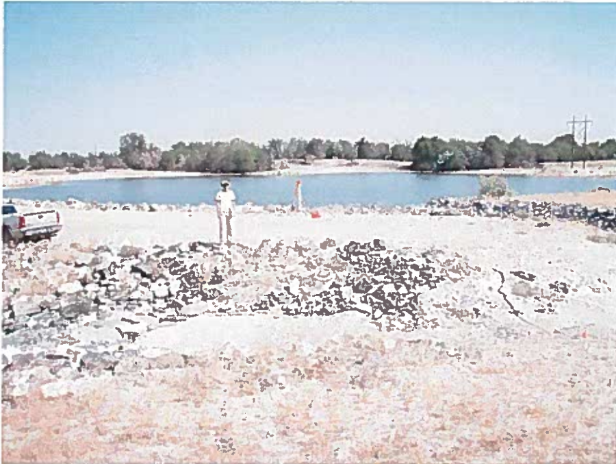
Figure 1: Malad Reservoir from southwest looking north east (2008)
