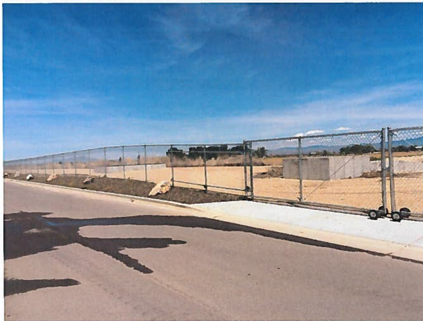
Figure 8. Turnout for surface water supply from Pioneer Irrigation District is located across school access road, southeast of track and northeast of well
