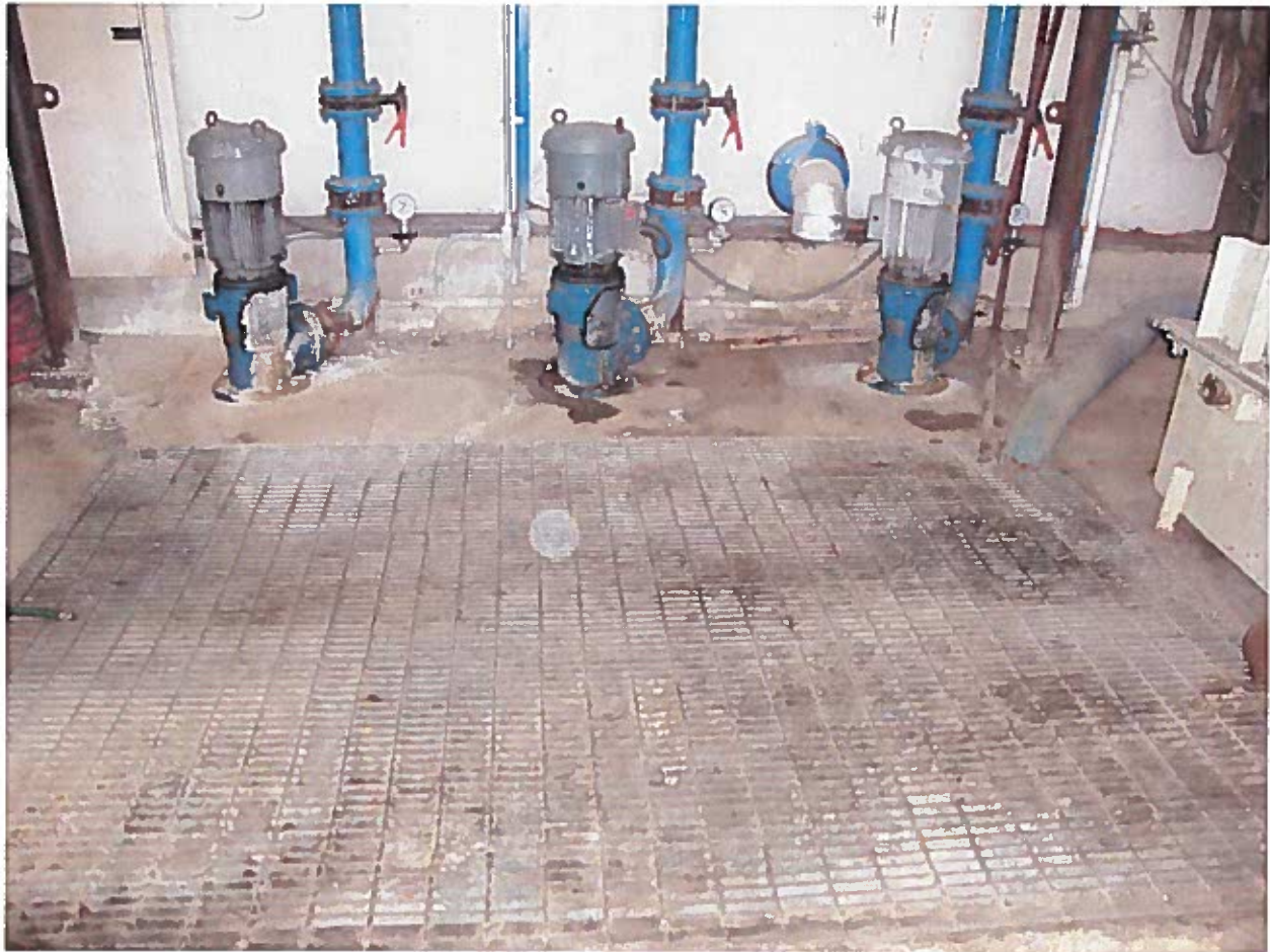
Above: Looking at the wet well sump.
