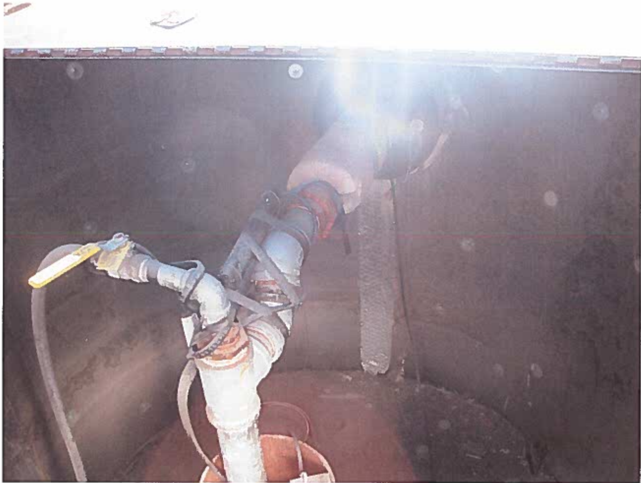
Above: Looking inside one of the culverts at the piping from the well that leads into the building.
