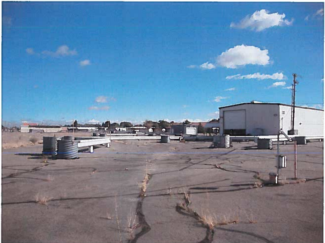
Below: Looking North in the SENE¼ of Section 25, T02N, R37E. The series of wells, protected by culverts.
