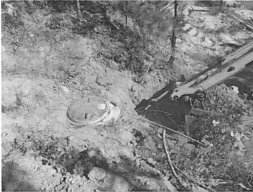
Beginning excavation of existing water tank.
