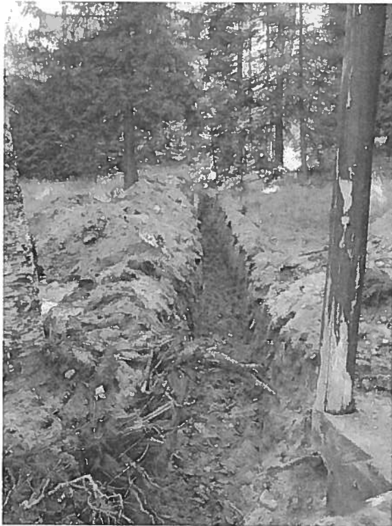
Utility trench in progress. Terminating at Cabin porch. Prior to hydrant installation
