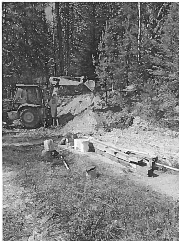
Final backfill being placed at new tank.
