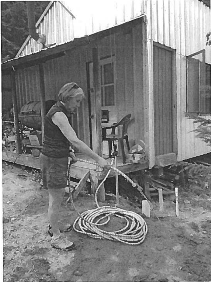
Water from new hydrant at cabin
