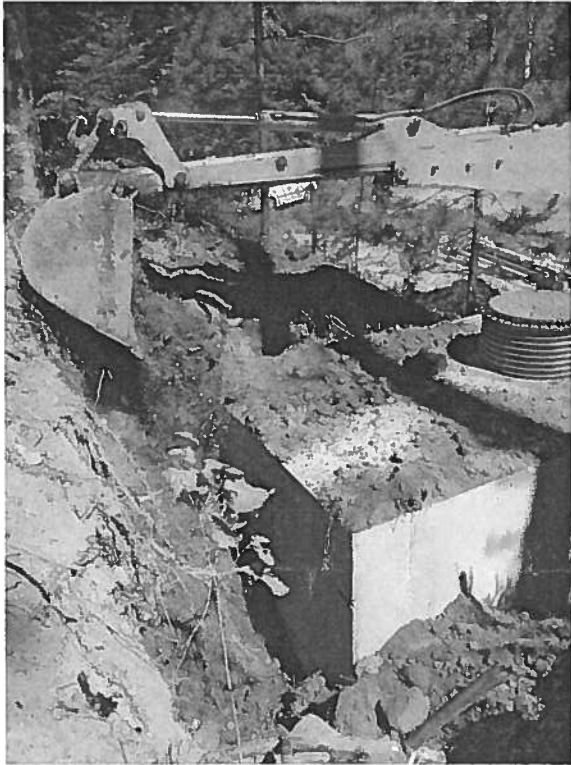
Backfill at new tank underway
