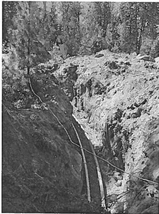
Utility trench showing water line and electrical conduit. Photo taken looking uphill toward existing house pad and existing tank location.
