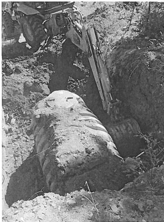
Existing water tank exposed ready for removal.
