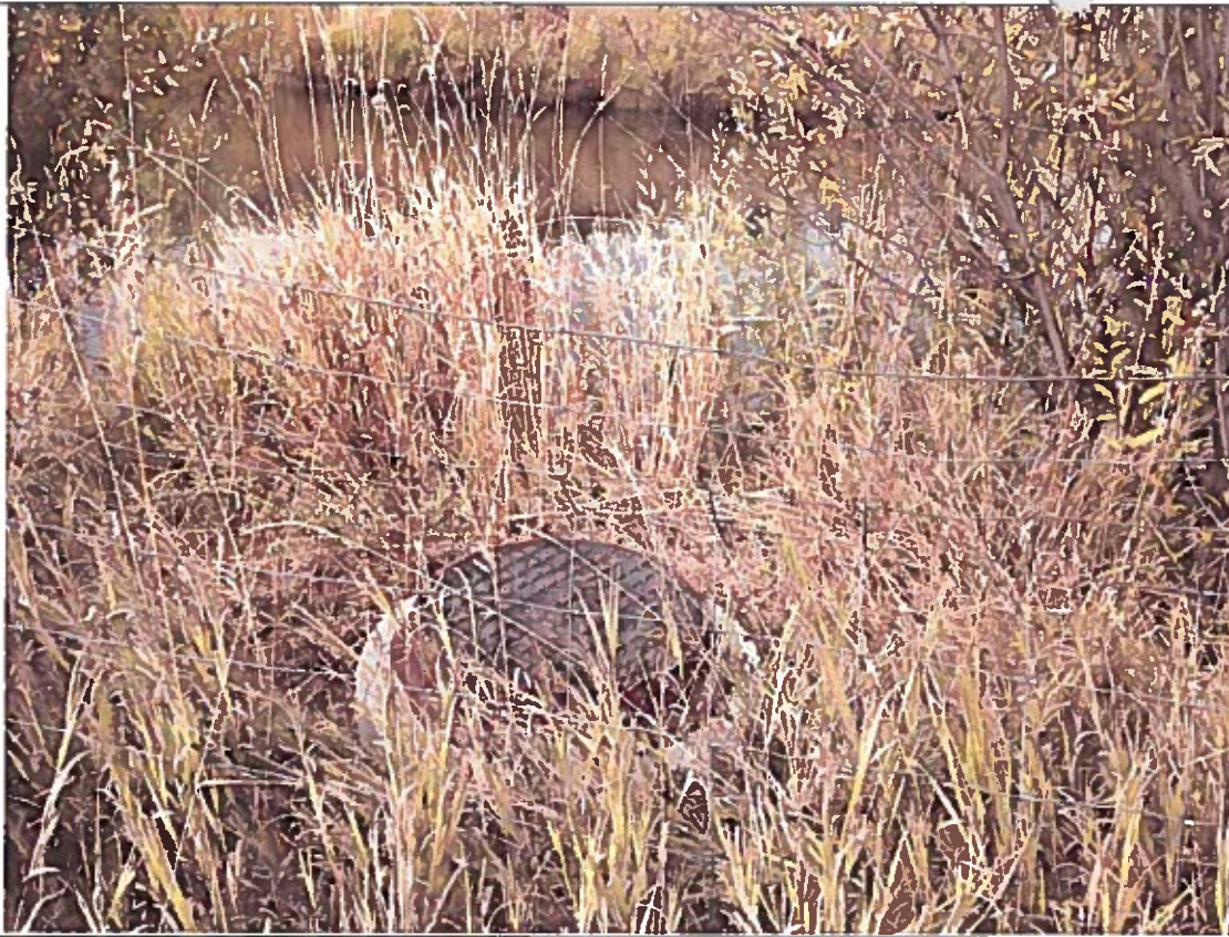
View of culvert showing its location on the banks of the Middle Fork of the Payette River
