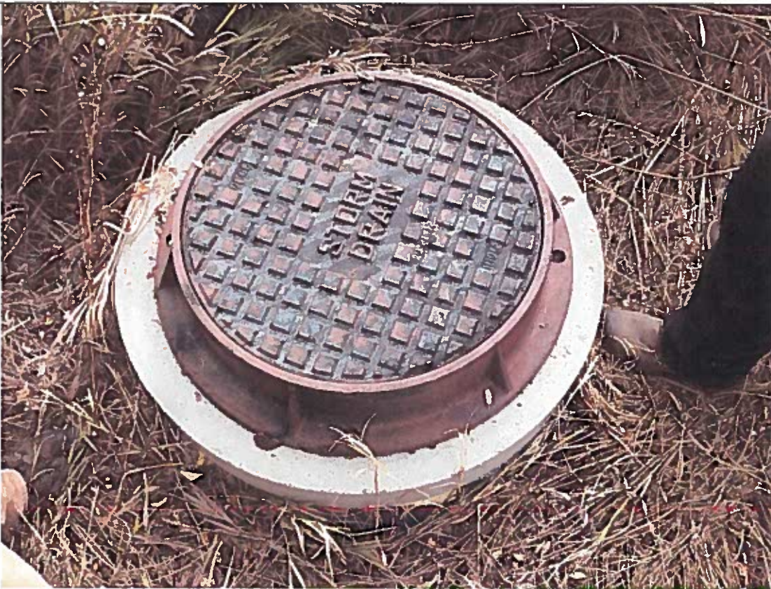
Top view of culvert with lid on
