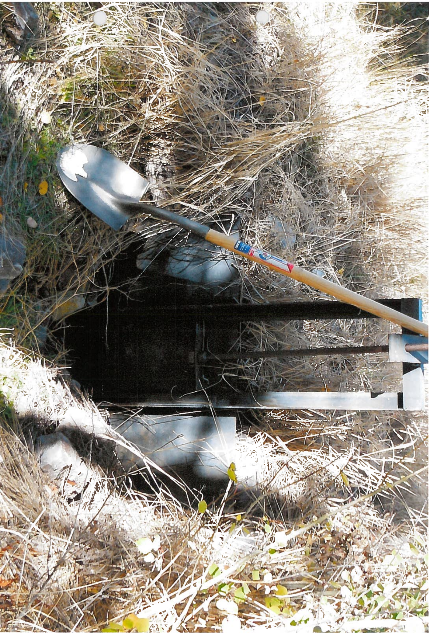
Peterson Creek Headgate October 8 th , 2015
