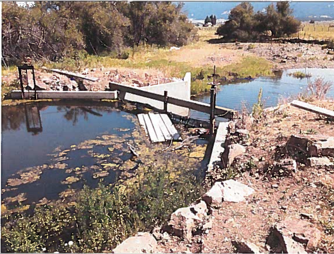
Diversion dam on Little Salmon River
