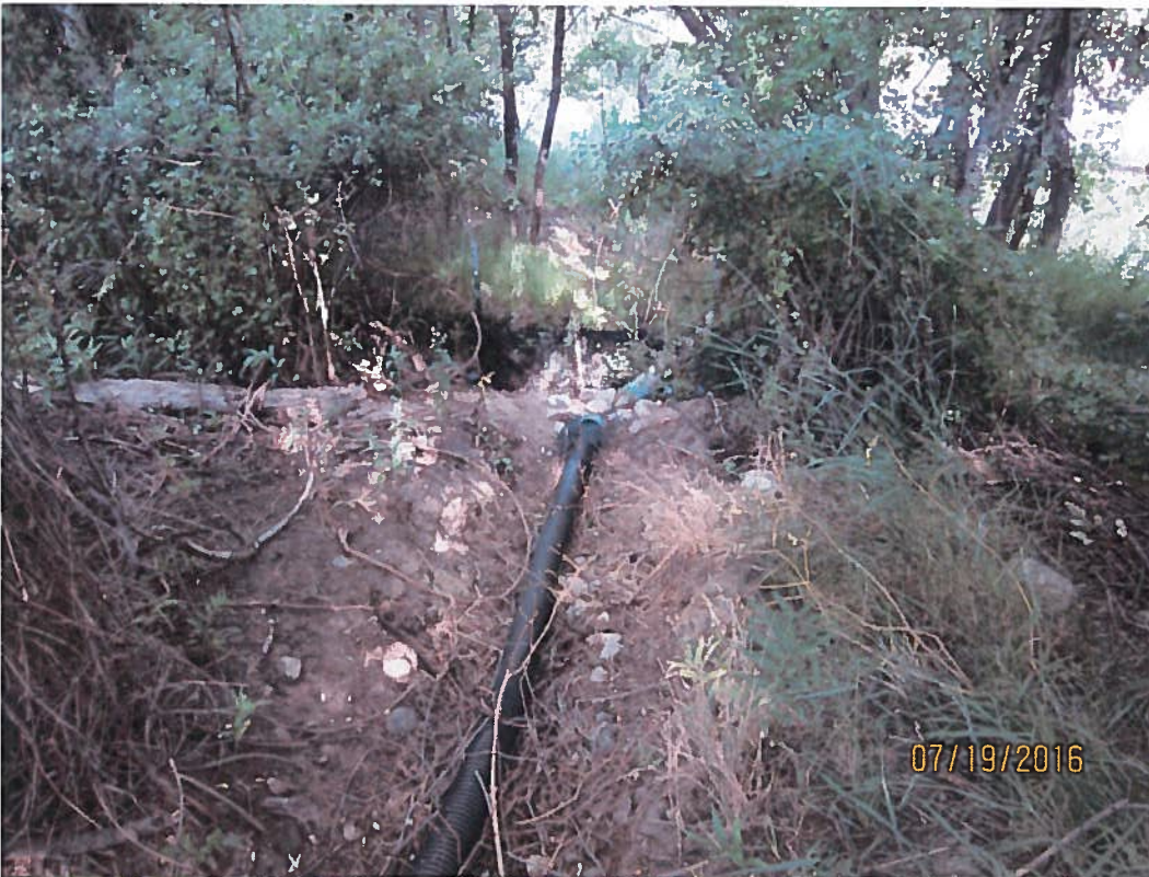
The top photograph shows the pipe that originates at the ditch.
