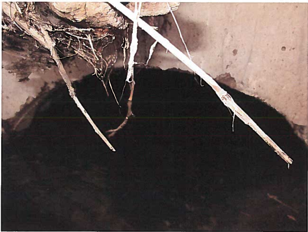
Above: The bottom of the 24" culvert that acts as the fish ladder around 6X diversion dam.
