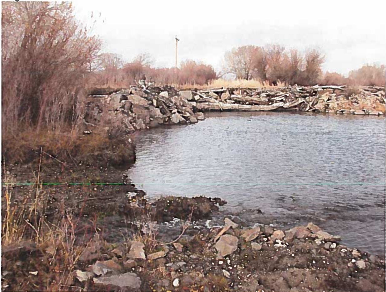
Below: 6X diversion dam in the background, with the stream outflow from the fish ladder in the foreground.
