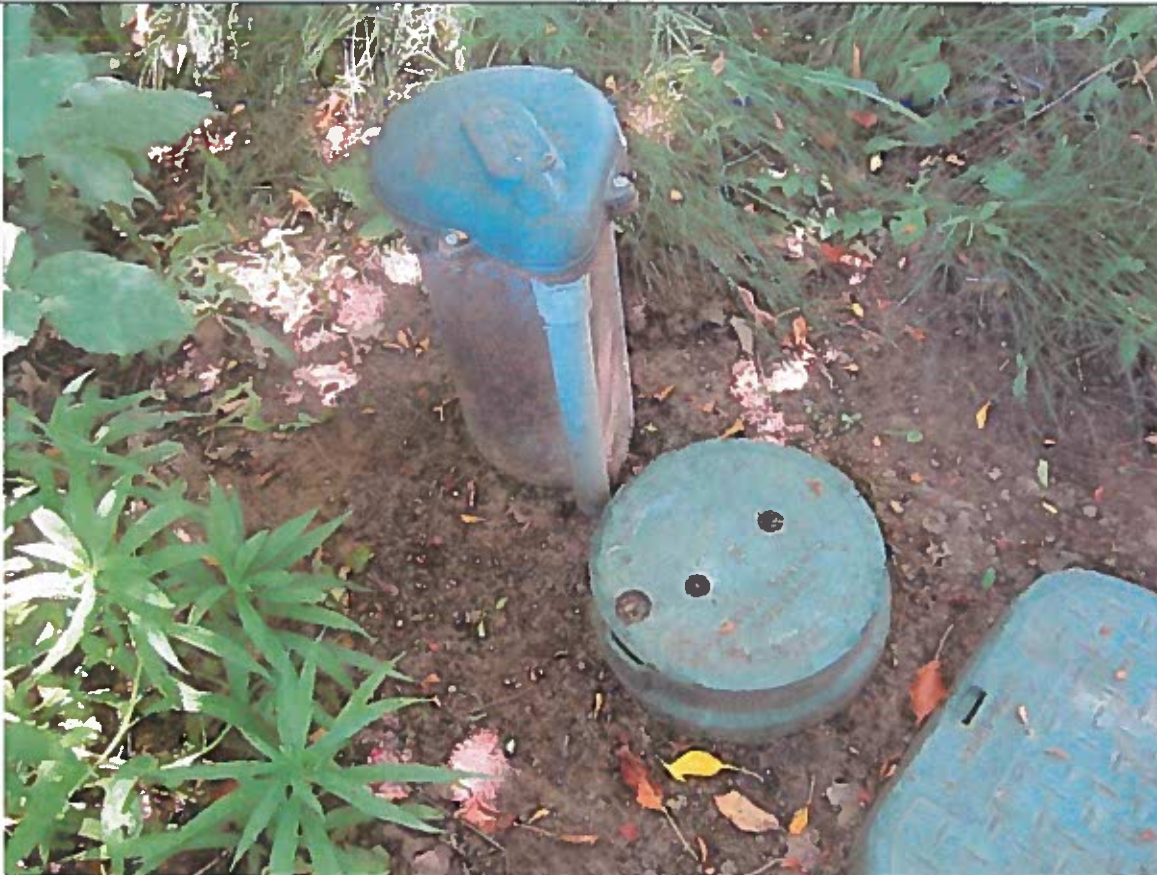
Looking southeast towards the well head
