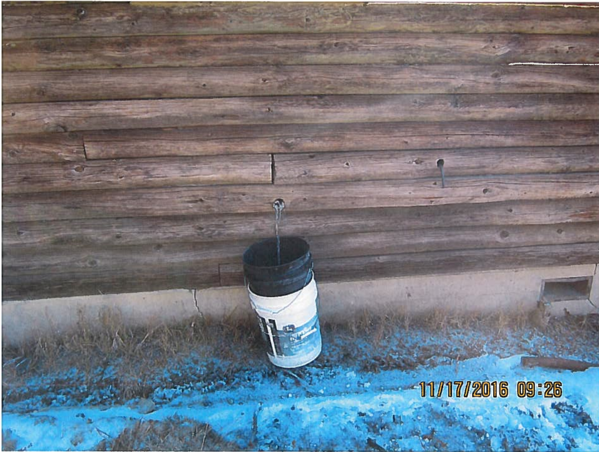
78- 12396 Goose Lake Rider Cabin POU Outflow pipe
