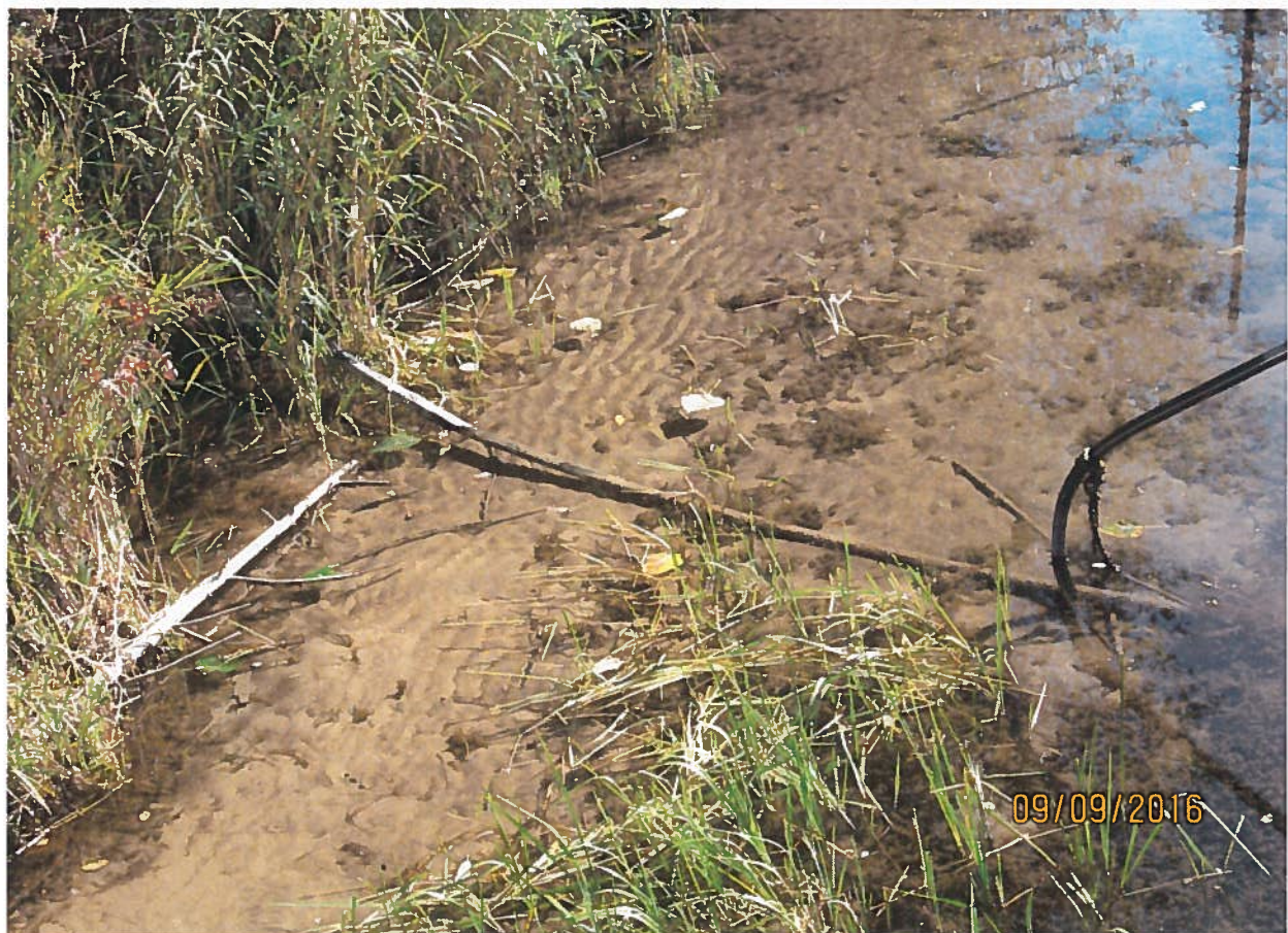
Intake line from river to shore.
