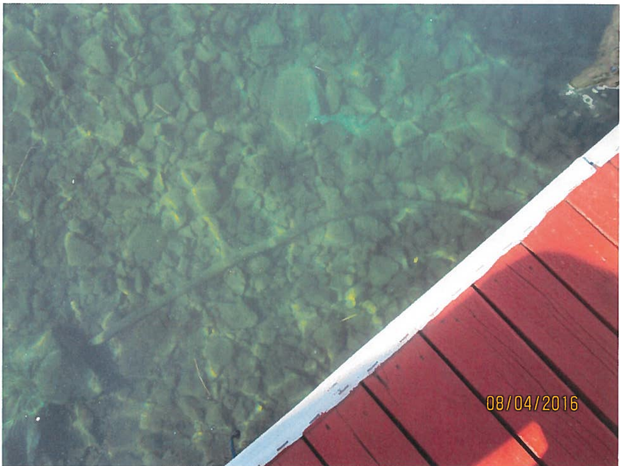
Intake line in lake.
