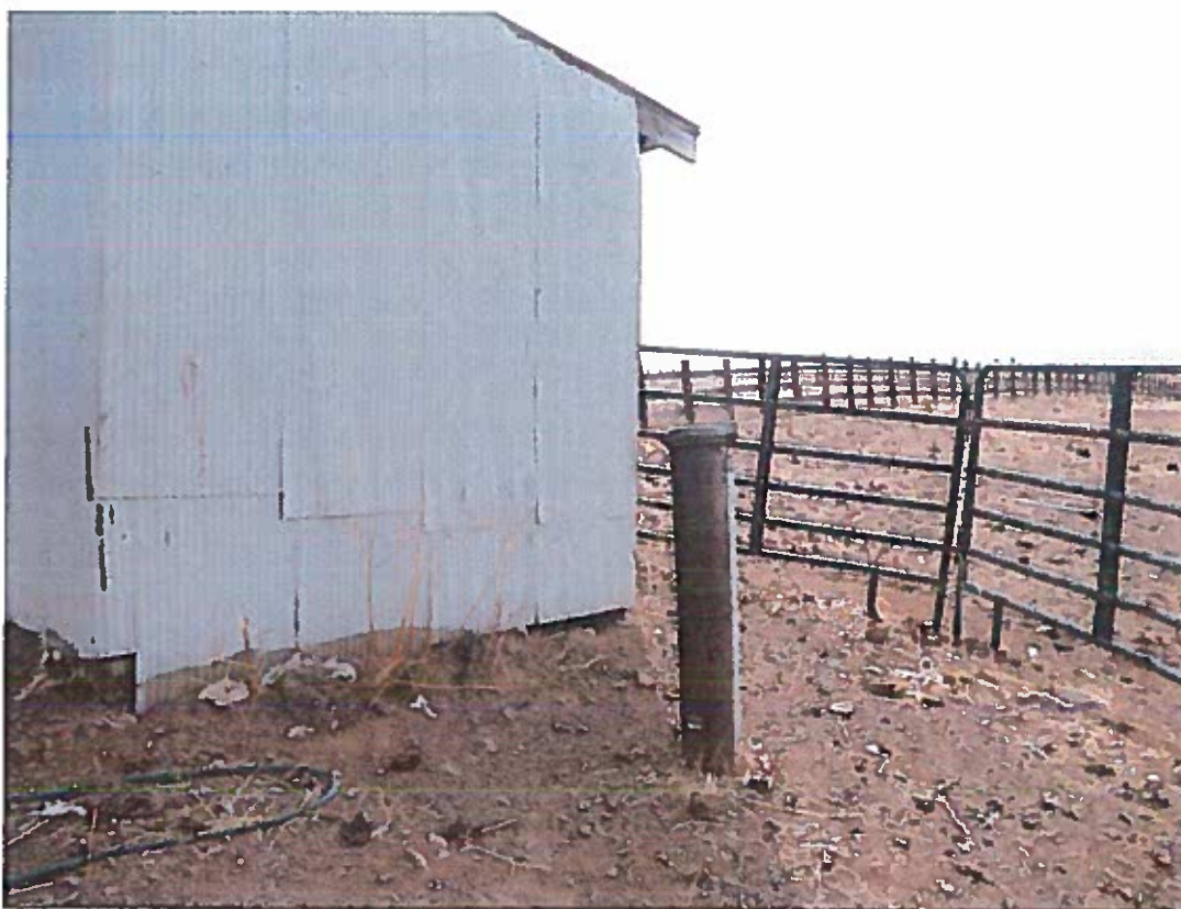
67-14250 Site Visit 9/23/2014: POD Stockwater well D0030795.
