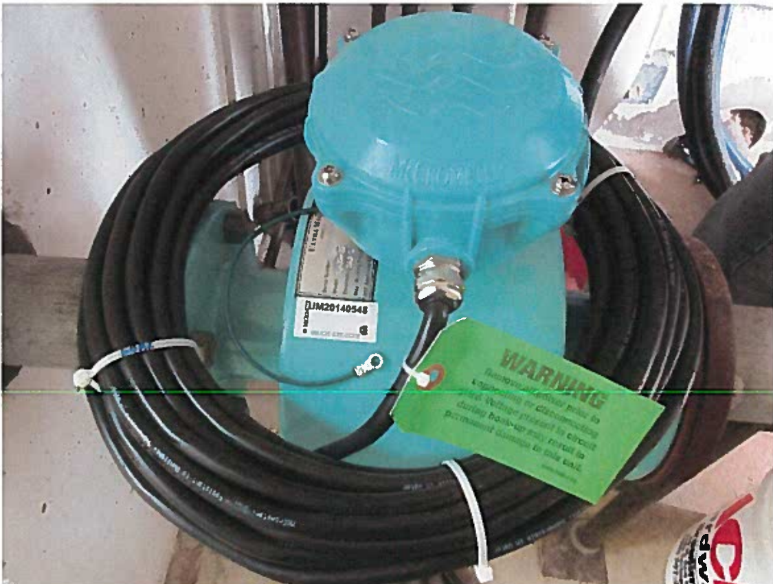
New flow meter being installed
