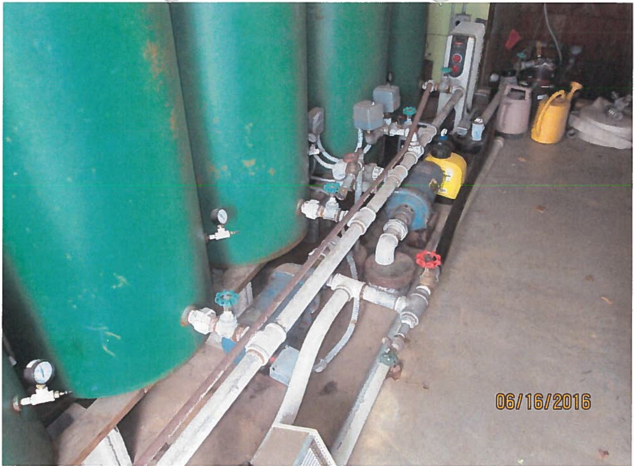
Pressure tanks and pump from storage tank.
