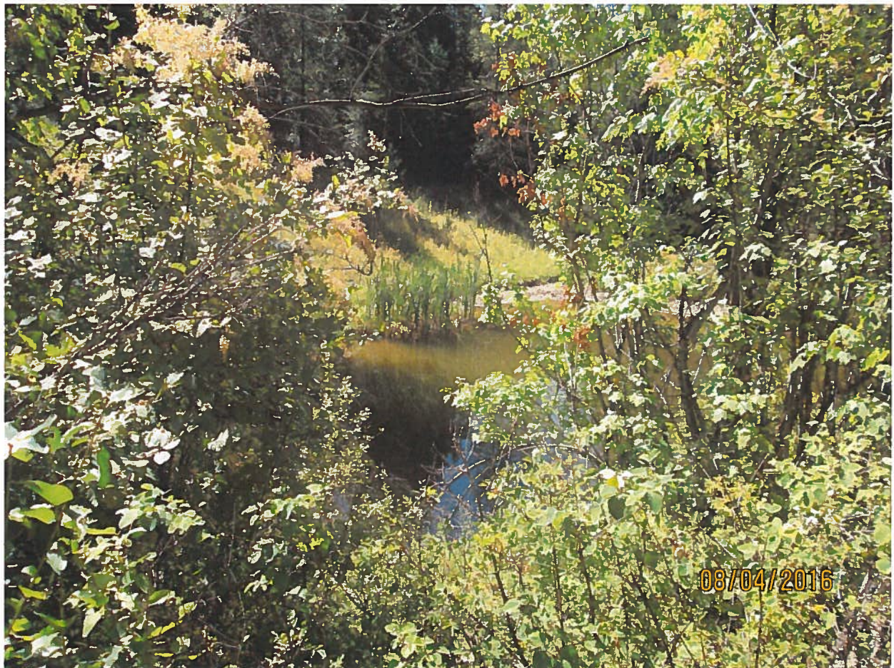
Looking at pond towards dam.
