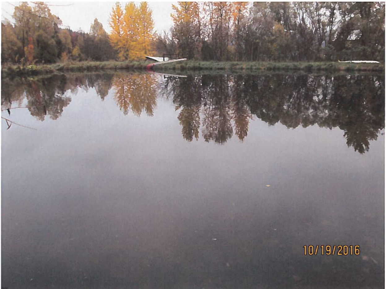
View of dam, on left side is overflow back into Alder Creek.
