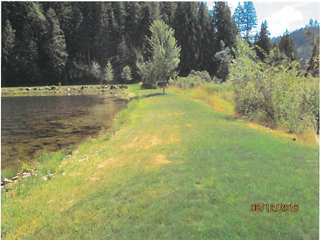
Looking at dam from driveway towards outlet culvert.
