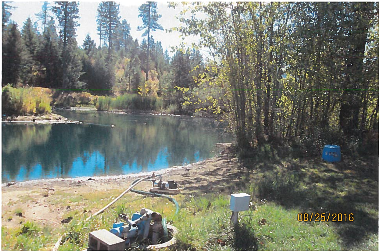
Stilling well adjacent to pond. 2 hp pump to irrigation.
