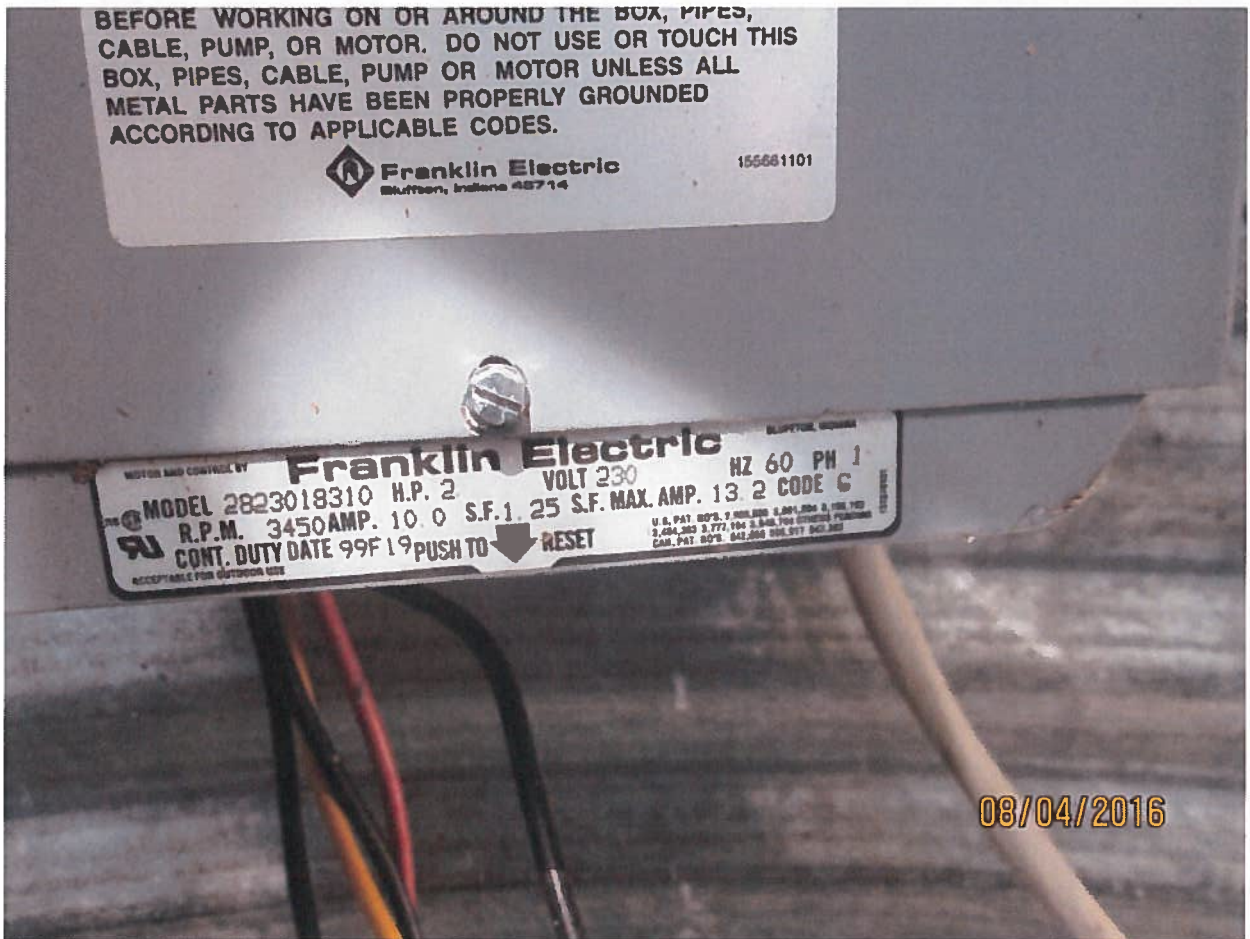
2 HP pump in well drilled by Arnold Sharp to 225 feet. Assumed pump set at 210 feet.
