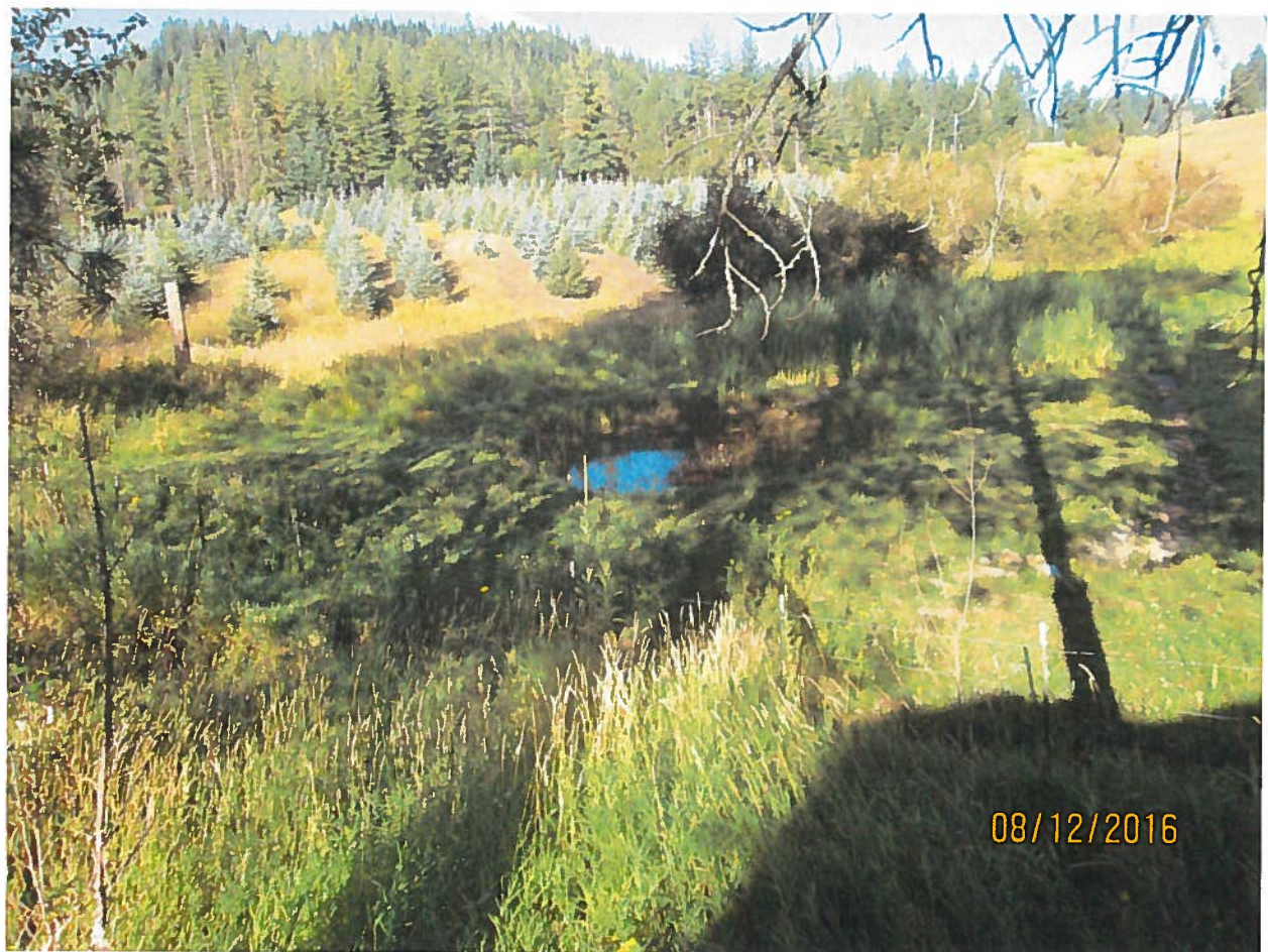
View of pond from dam looking uphill towards source of water.
