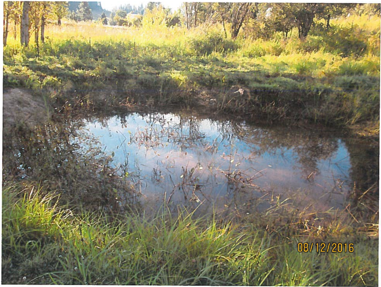
View of dam.
