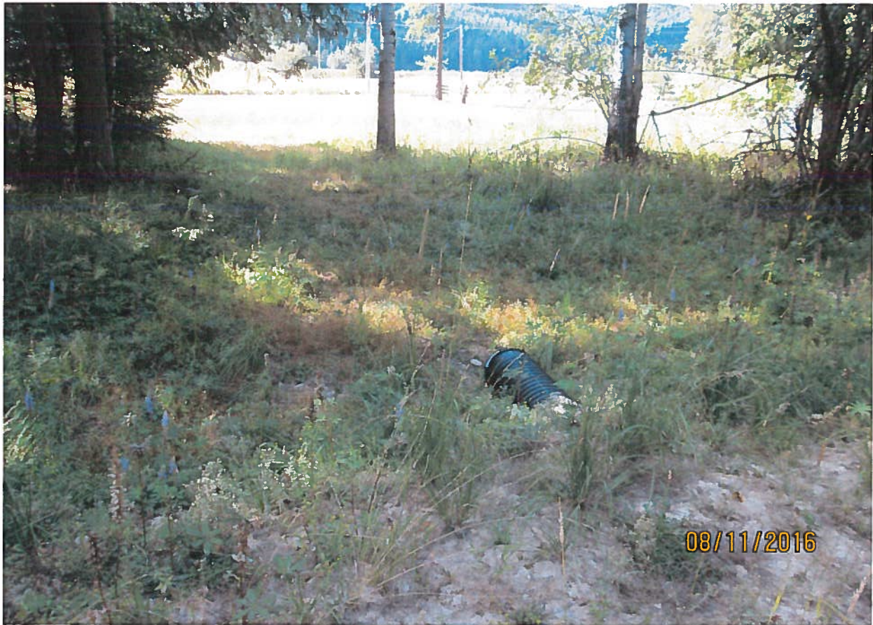
Looking below dam at overflow culvert 1.
