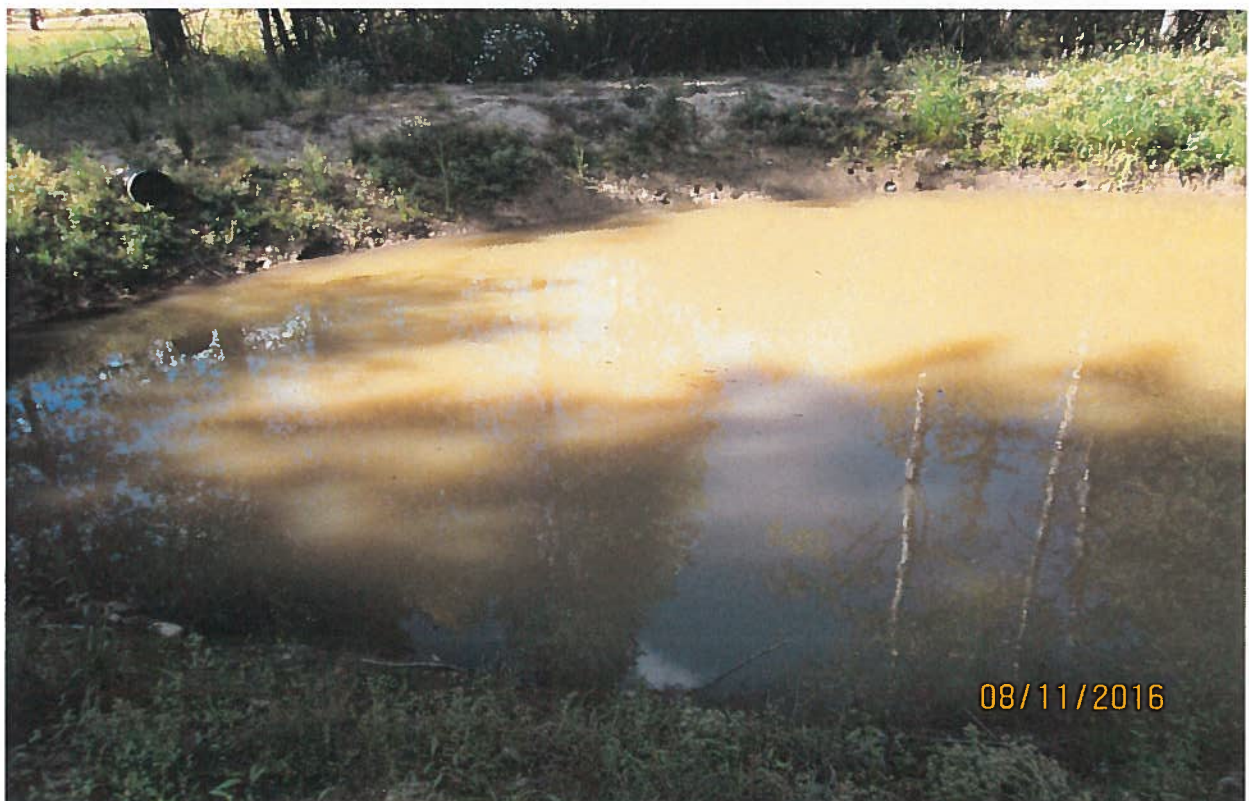
Looking at dam from driveway towards culvert 1.
