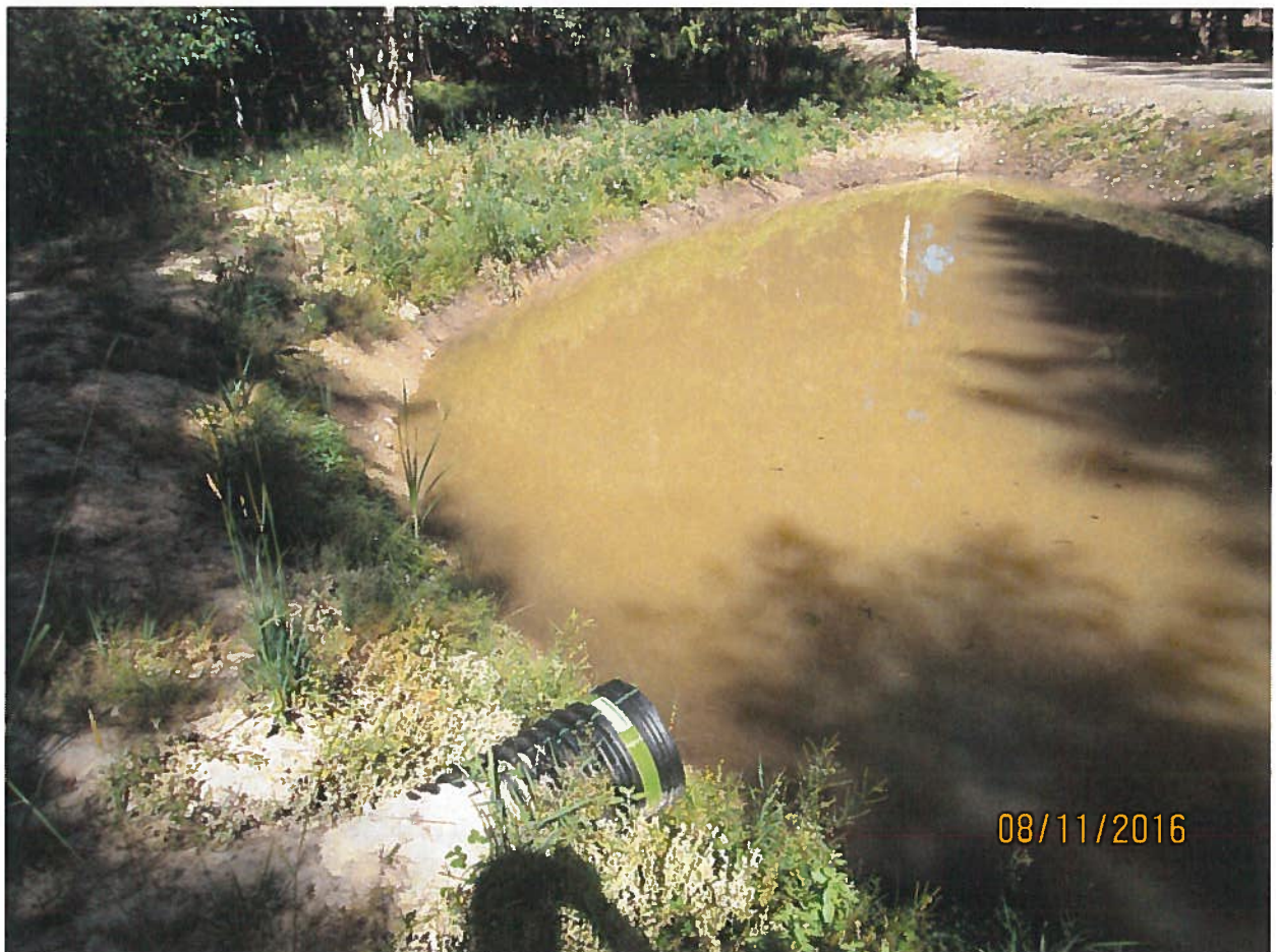
View from 6 foot high dam. 1 of 2 overflow culverts below.
