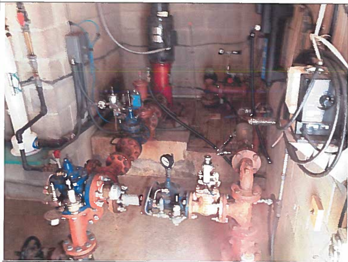
Inside Pump House.
