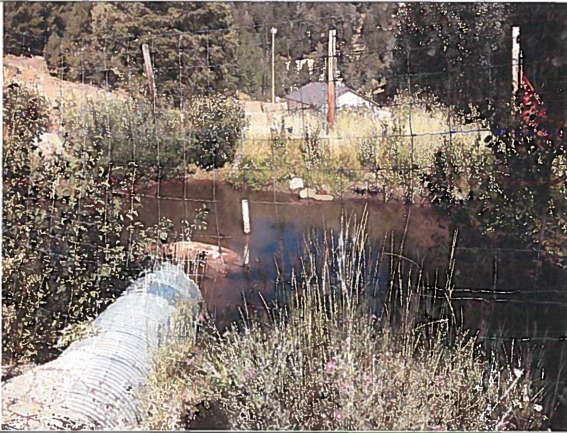
Bogus Creek enters small pool through large culvert above sand filter (shown in distance).
