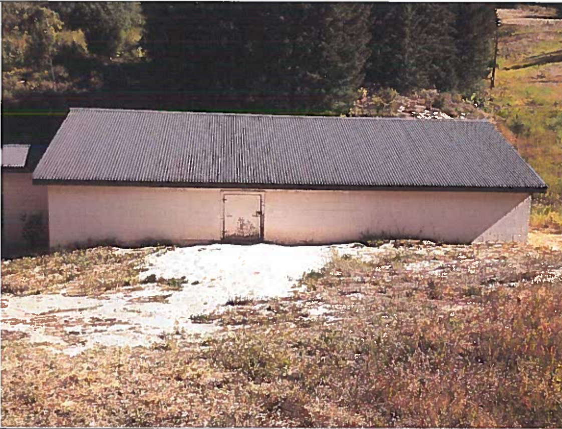
Sand Filter House
