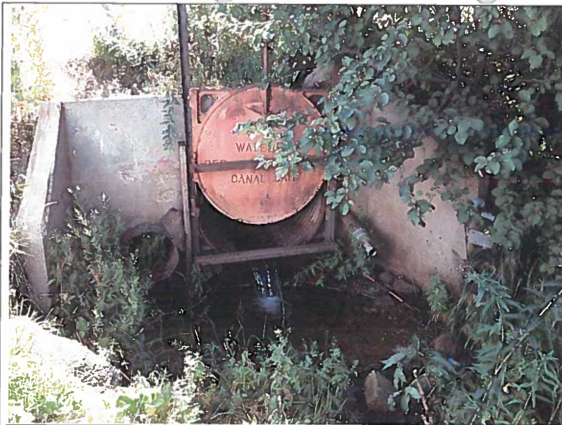
Bogus Creek at Pump House location.
