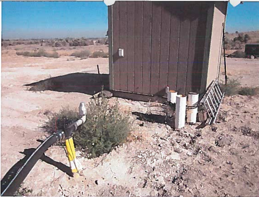
5. First riser connecting well to lots 3 and 4.
