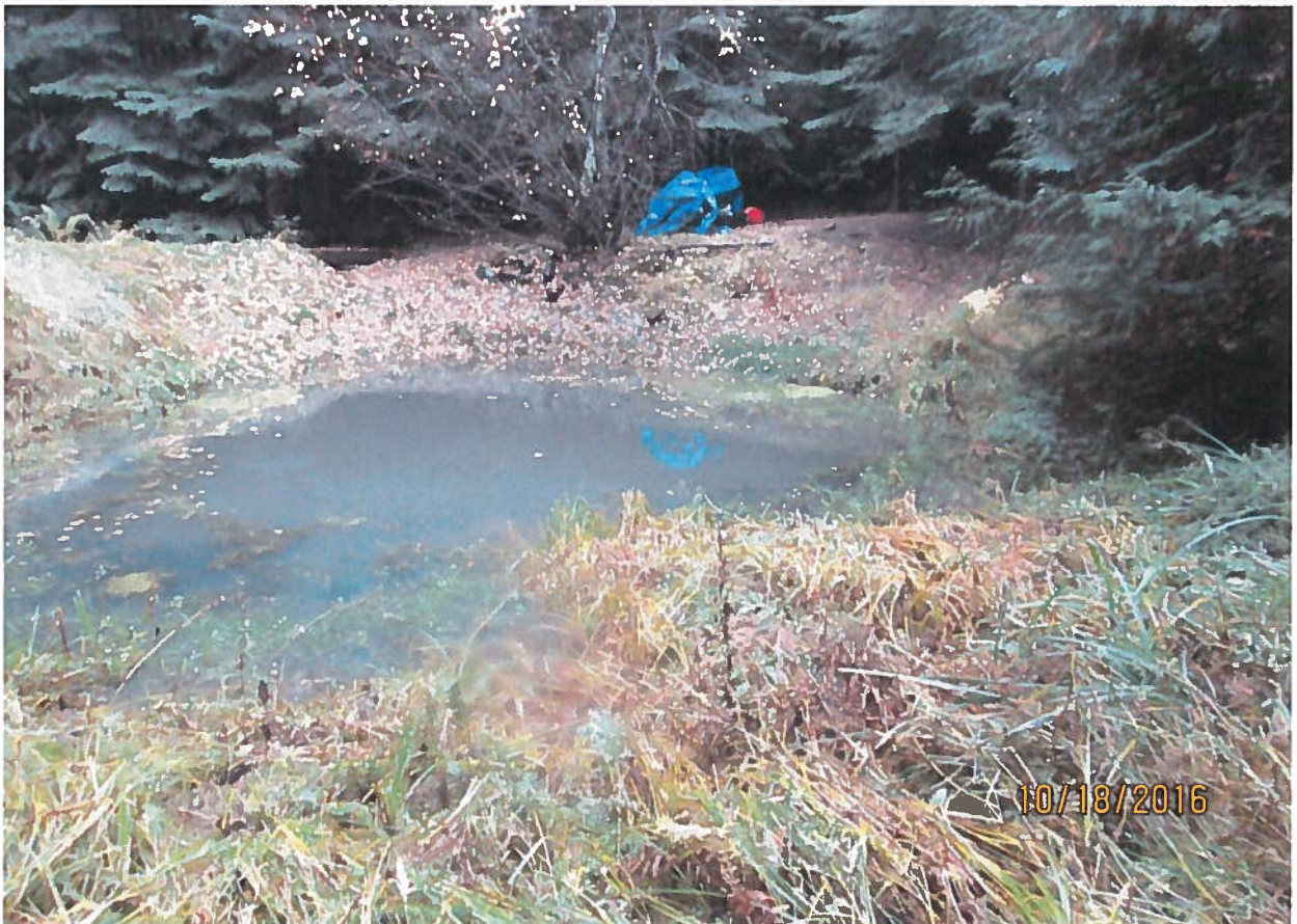
Pond looking back towards spillway.
