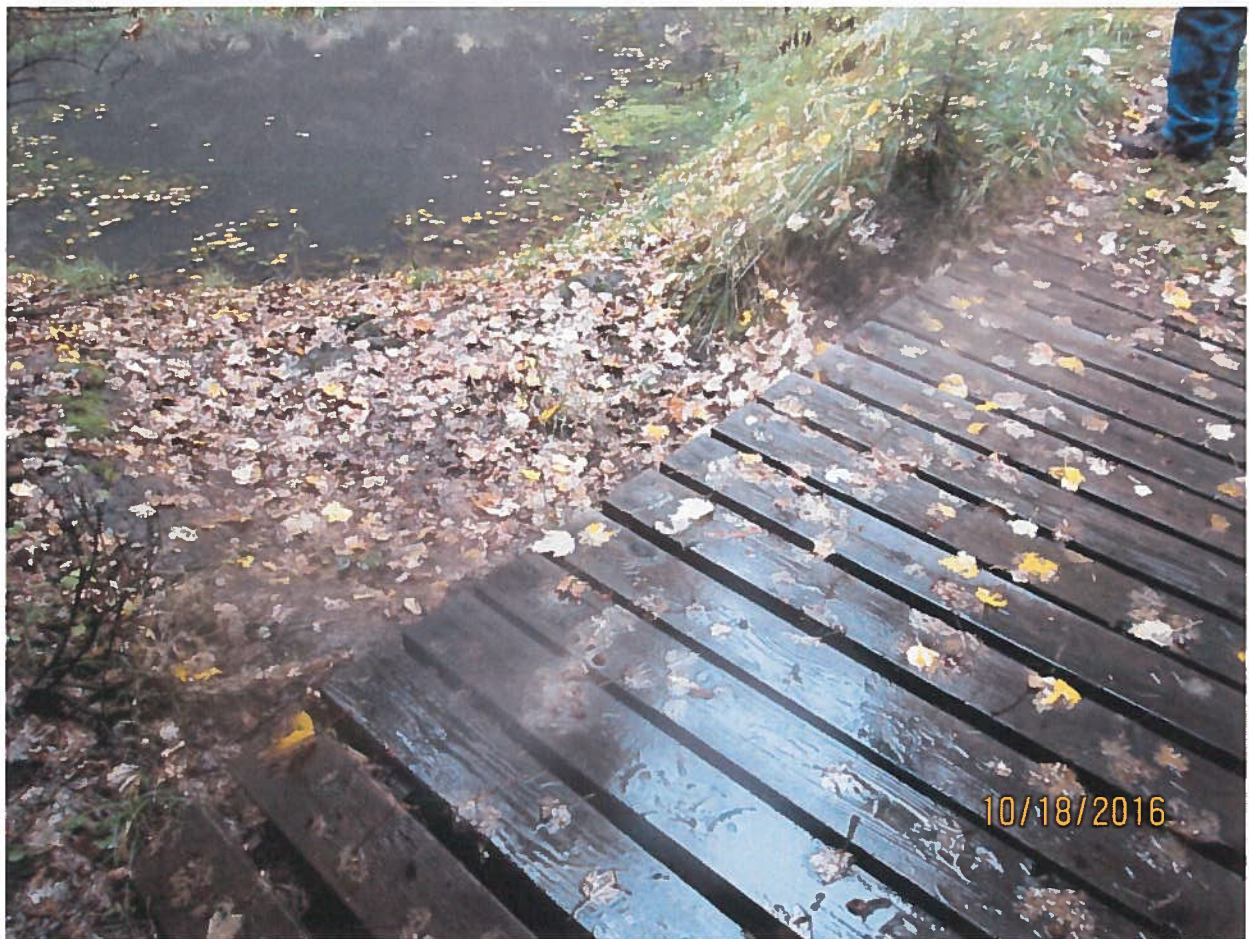
Spillway for water to overflow and continue down unnamed stream.
