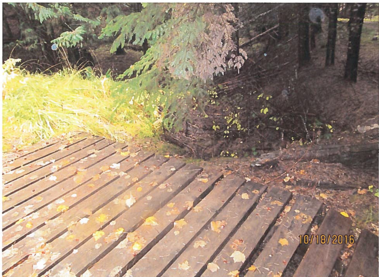
Unnamed stream below spillway.
