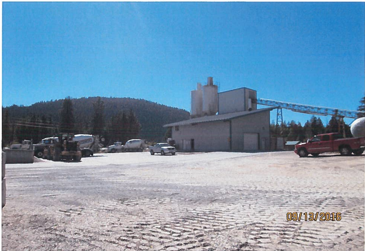
Place of use, concrete plant.
