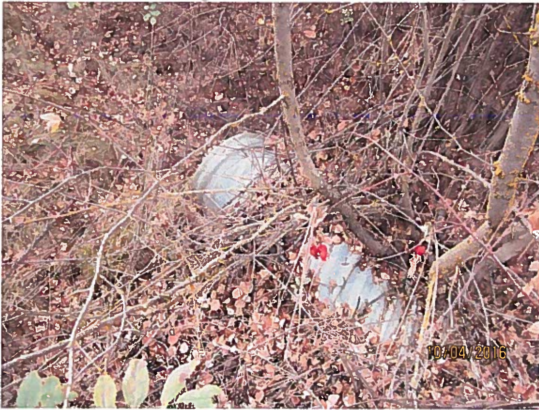
Corrugated pipe along Middlefork Road that delivers water to the unnamed stream.
