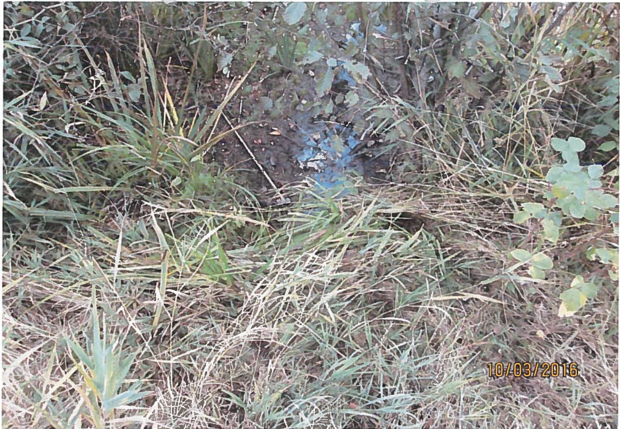
Culvert under road leading into pond from unnamed stream.
