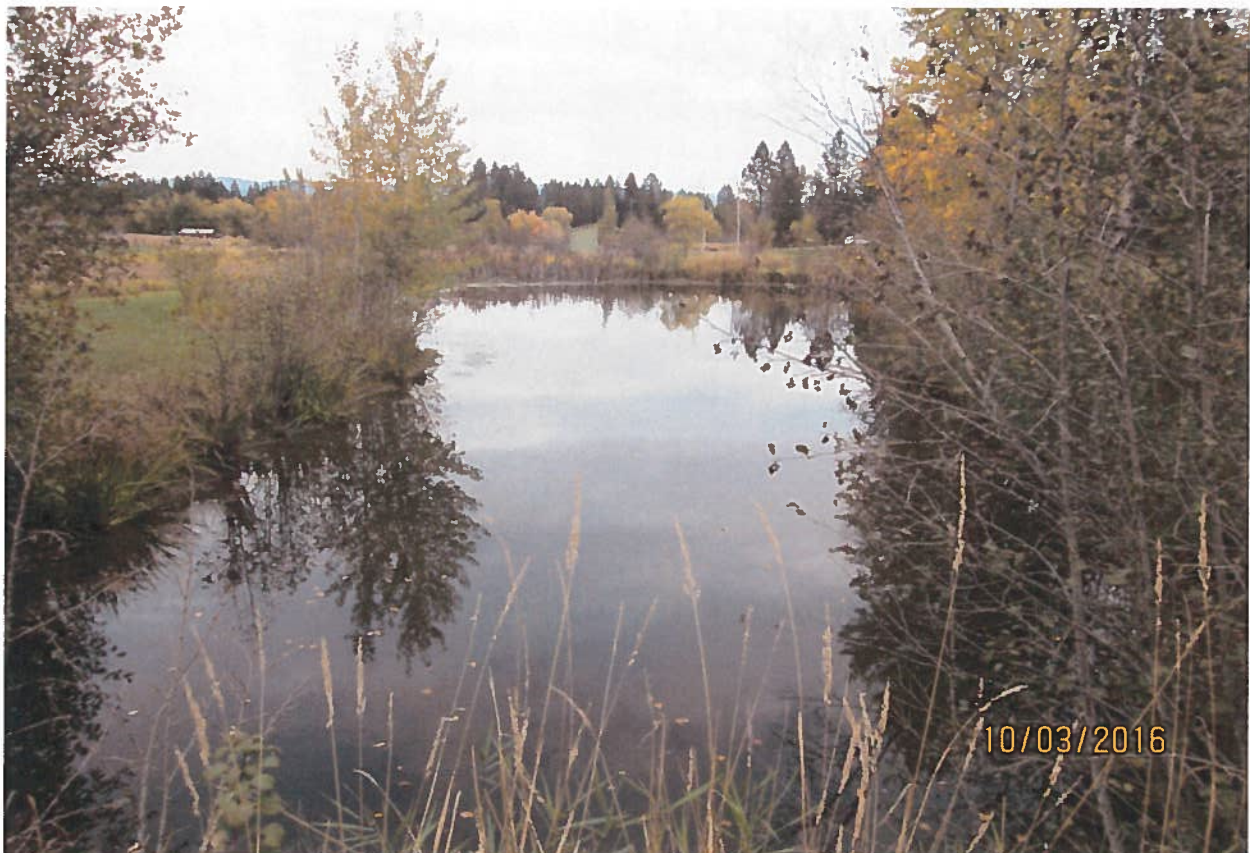
View from roadway looking towards dam to west.
