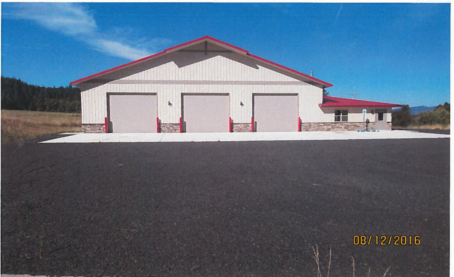
View of fire station.
