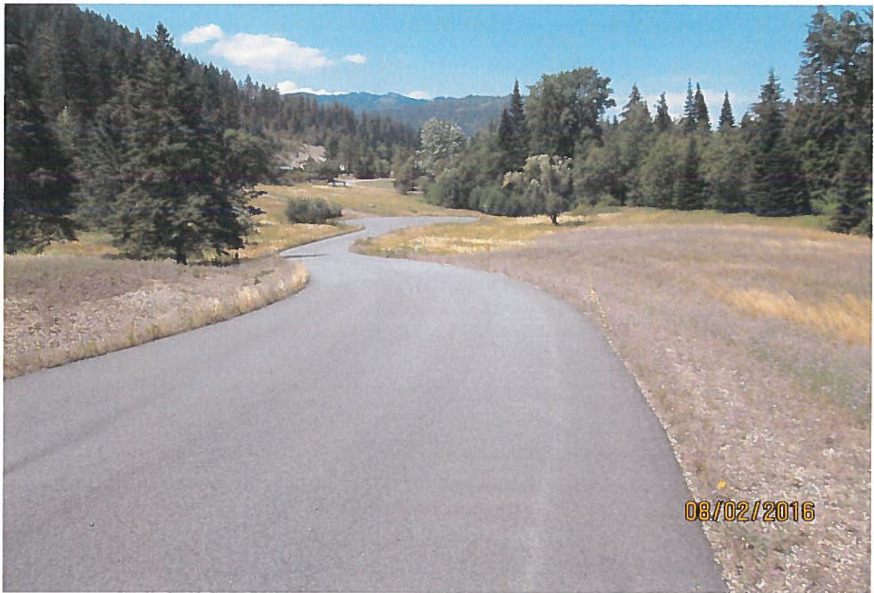
Sub division road.
